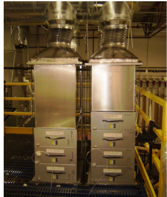
Figure 1: Full size testing showing two sets of filters at Entegris' Franklin, MA facility during a performance test.
